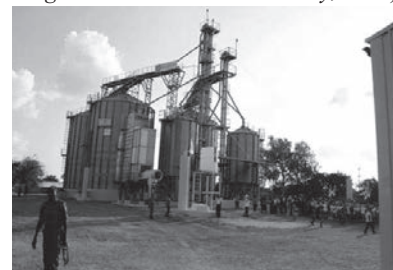
Fig. 6 Metal silos for postharvest maize storage (Source: Ministry of Agriculture and Food Security, 2015)
