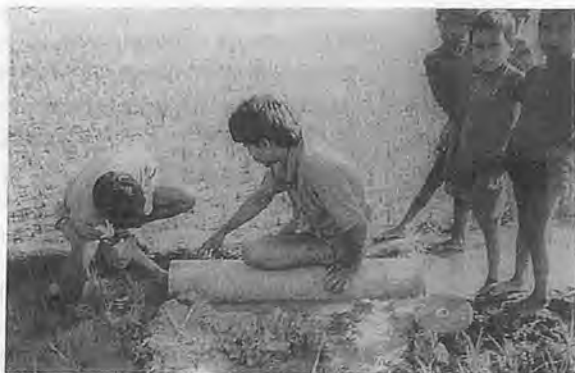
Fig. 2 Setting delivery pipe at the entrance of the field.
