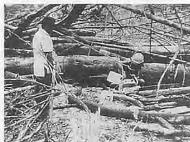
Fig. 3 A CSB cleared plot with logs being cross-cut.
