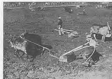
Fig. 3(a) Pond construction process by peasant associations using draft animal power.
