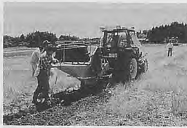
Fig. 9 Construction of underground drainage.
