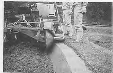
Fig. 5 Construction of levee covered with soil-mortar.
