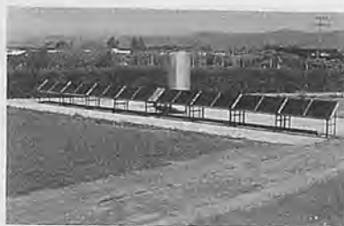
Fig. 4 Solar grain drying system.
