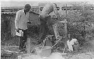
Fig. 2 Evaluating the performance of the manually-operated irrigation pumps.
