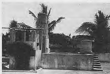
Fig. 7b Concrete soaking and steaming tanks (Side view).
