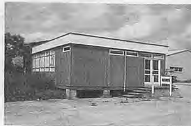
Fig. 2b The experimental building.
