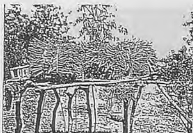
Fig. 7 Typical platform structure.
