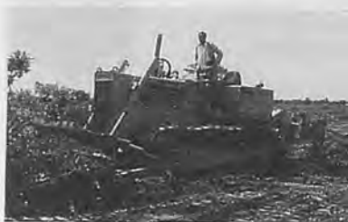
Fig. 1 Bulldozing of top soil by crawler-type tractor.
