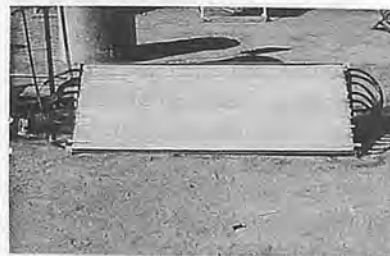
Fig. 1 Natural solar water heating system made of concrete materials.
