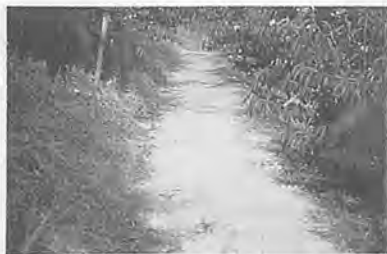
Fig. 8 Paved branch road with coagulator.
