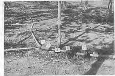
Fig. 4 Assembly of fittings in a bamboo drip irrigation system.
