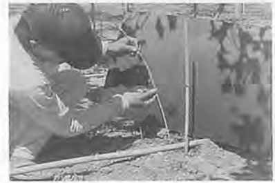
Fig. 9 Cleaning of algae infested low-cost emitter in the field.
