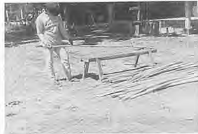
Fig. 2 Making of bamboo pipe.
