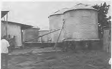
Fig. 8 Aluminium silos for storing grains in Western Nigeria.
