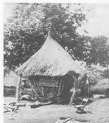
Fig. 3 Nigerian local storage structure with inadequate facilities or provision for quick drying.
