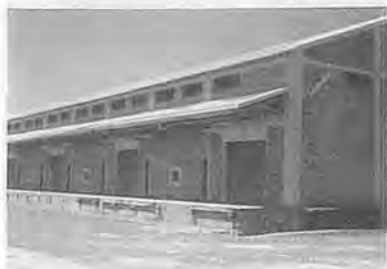
Fig. 7 A row of warehouse in the Food Corporation of India, Borovli, Bombay, India.
