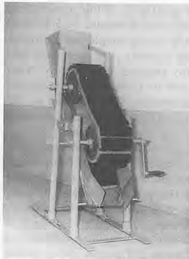
Fig. 3 The ginger peeling machine developed in the study.
