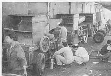
Fig. 7 Modified dual-mode all-crop threshers being commercially produced by one of the cooperating AMRI manufacturers in Tanta, Egypt. AK 1990.
