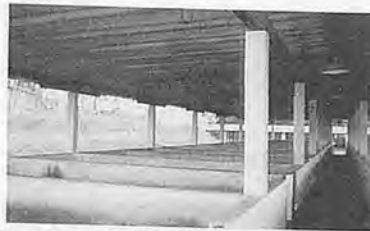
Fig. 2B Inside view of the studied Brazilian swine building.
