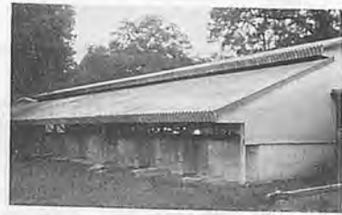
Fig. 3A Front view of the studied American swine unit.
