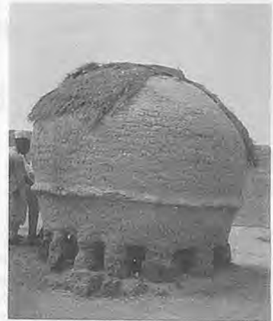
Fig. 2 Mud rumbu structure in Kaduna state. Capacity: 3 t.
