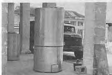
Fig. 6 Metal bin. Capacity: 1000 kg.
