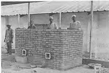
Fig. 8 Indoor brick masonry structure (under construction). Capacity: 2 t.
