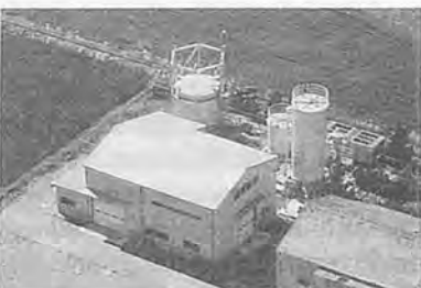
Fig. 6 Rice husk gasification and utilization system
