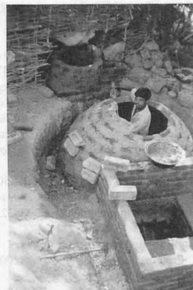
Fig. 3 Konark model biogas plant under construction.
