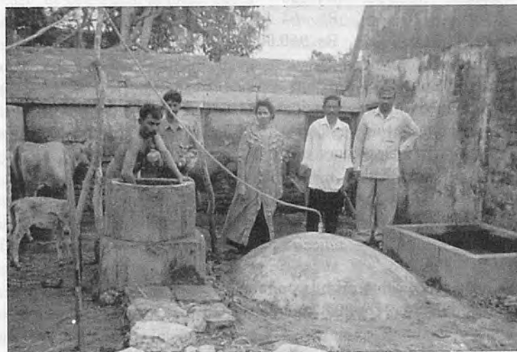
Fig. 4 Beneficiary mixing cow dung with water in the mixing tank of Konark biogas plant.
