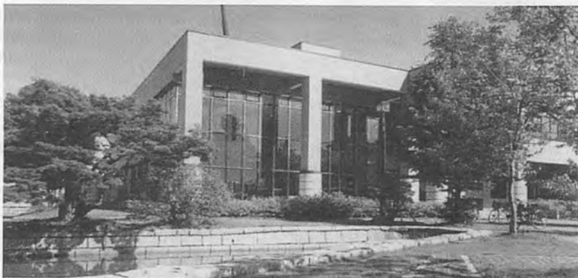
Fig. 3 Library building at Ami Campus.
