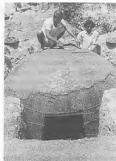
Fig. 6 Construction of Utkal model bio-gas plant.
