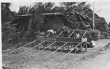
Fig. 3 Dryer under construction
