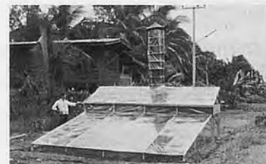
Fig. 4 The completed dryer
