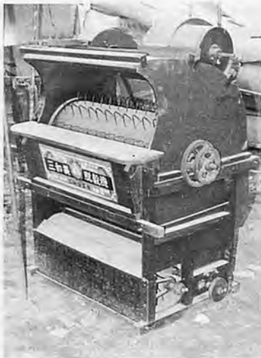
Fig.3 A small low-cost drum-type thresher still being developed by a Korean small shop for sale to individual farmers.
