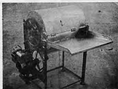
Fig.9 The IIRI Portable Thresher
