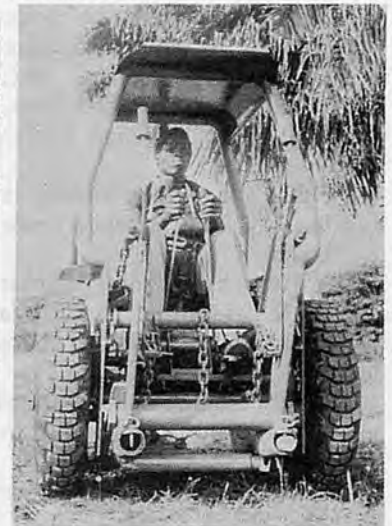
Fig.4 A Simple, Locally made Prime-Mover which is installed by village artisans
