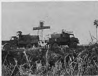
Photo.20 Truck tanks below top of elevator
