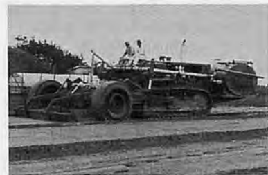
Photo.15 Asphalt barrier machine for sand dune field.
