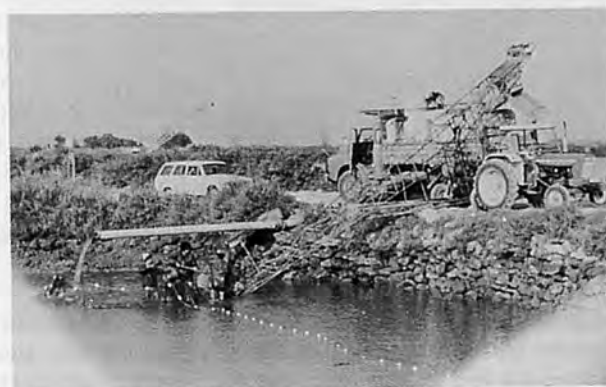
Photo.16 Loading the trolley
