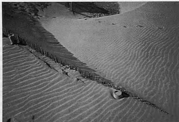
Photo.2 Protection for sand scattering.
