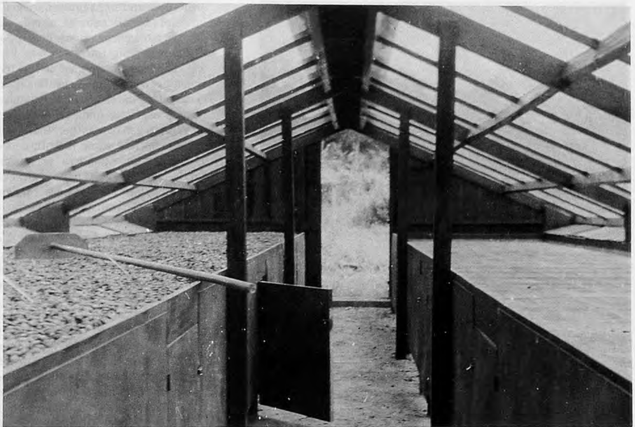
Fig.1. Glass-roof dryer—inside view.
