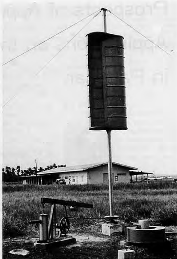
Fig.3. Savonius vertical axis windmill.
