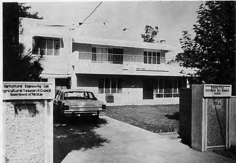
Fig.1. The office of Regional Agri. Mechanization Program IRRI, in Rawalpindi, Pakistan. The shop is located on the back of office building. The adaptation of IRRI thresher to suit local condition has been completed. The thresher marketability has been increased due to its wide range threshing ability of all cereals i.e. wheat, rice sorghum, millets etc. The Power tiller Project is near to start.
