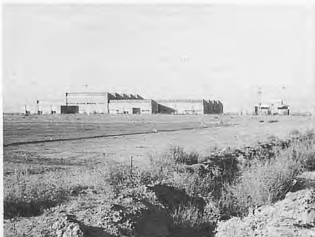
Photo.3. Iran. Large-scale comprehensive development project. Land Cultivation Service Co., Central Workshop & Head Office.
