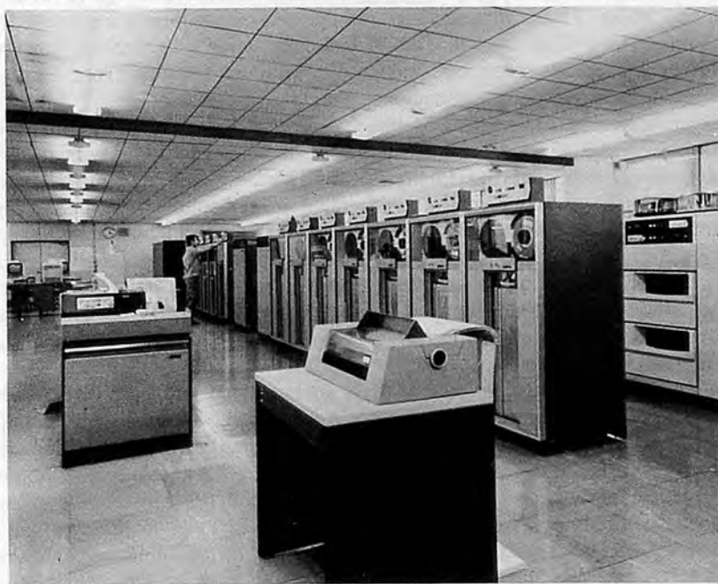
Photo.1. Computer center in head office.
