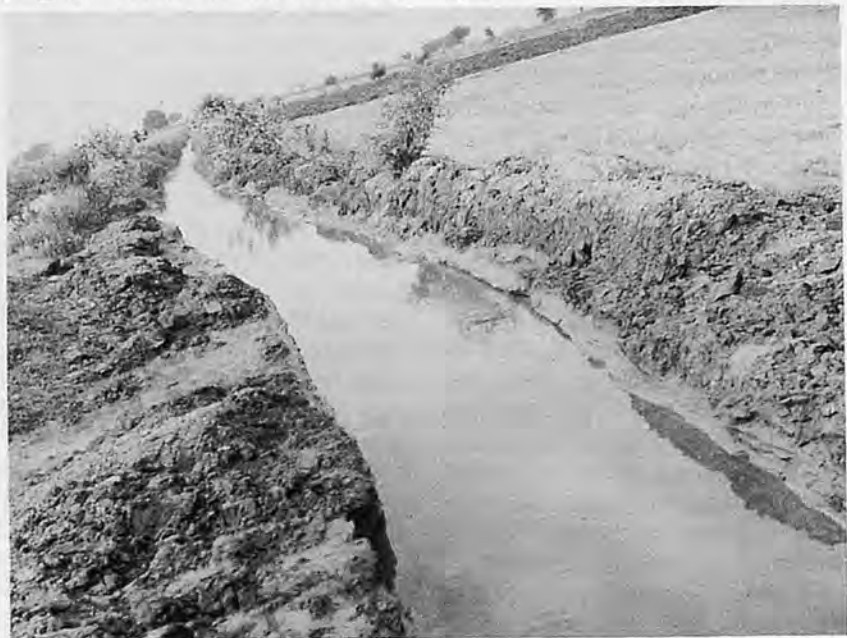
An unlined distributory of a canal irrigation system. Seepage forms the main source of water loss in irrigation projects. The loss may be as high as 25 to 40 per cent in a long unlined field water course in a sandy or sandy loam soil.
