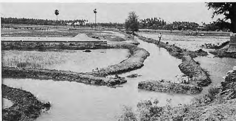
Inadequate drainage, poor field layout, high losses due to deep percolation, and inadequate irrigation at critical periods are the chief water management problems facing the low-lying rice growing areas.
