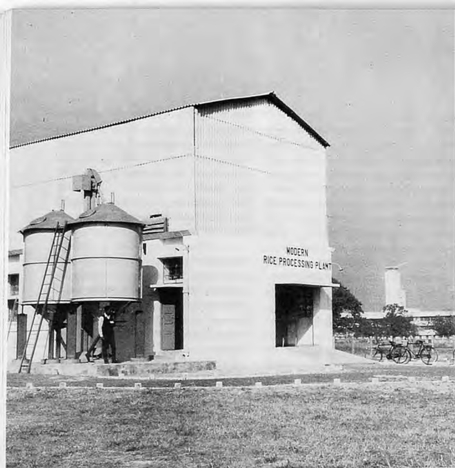
Modern rice processing plant (India)
