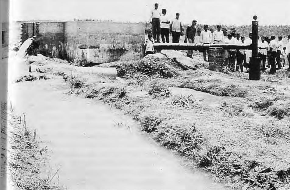
Fig.2 An artesian tube well discharging about 150 litres per second in the Terai region of the State of Uttar Pradesh
