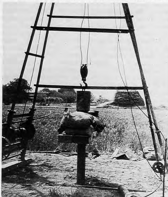
Fig.3 A manually operated percussion drilling rig for constructing shallow tube wells.
