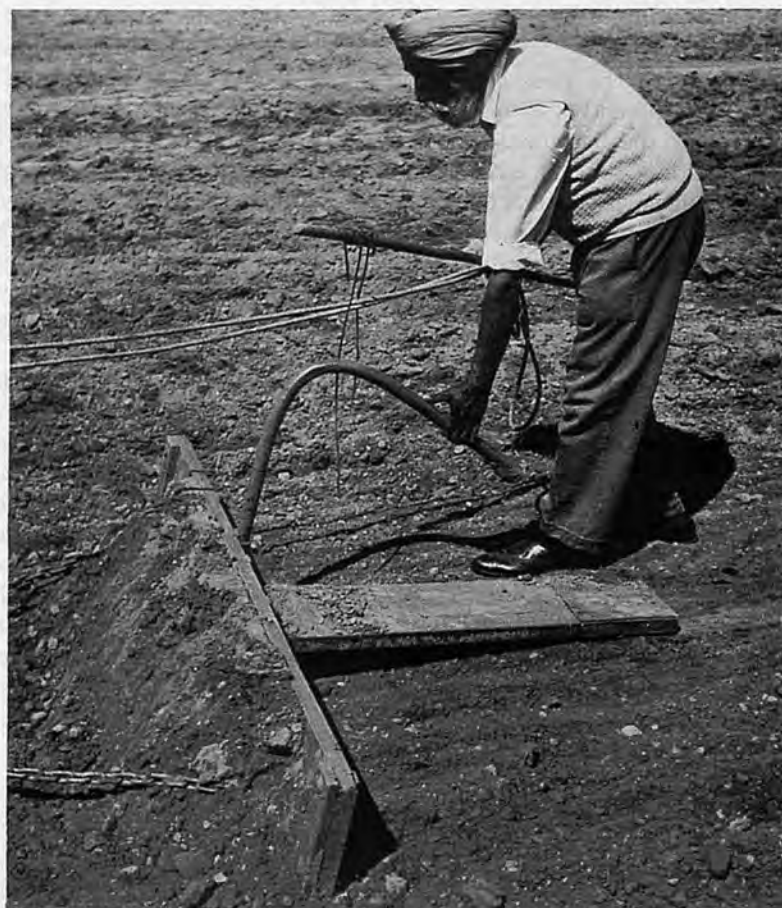
An animal-drawn buck craper used to grade land for efficient irrigation
