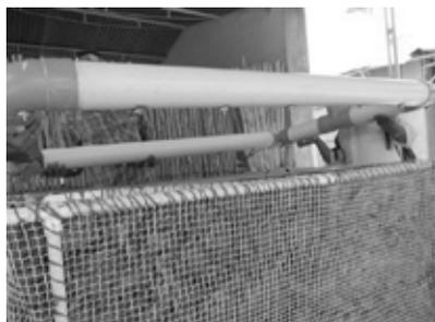
c. Dripper discharge over coconut cooling pad
