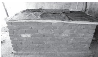
**Fig. 12** Evaporatively cooled storage structures used for storage of seed ginger.
