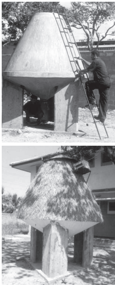
Fig. 5 Pictorial view of the bin after construction at the NERD Centre
